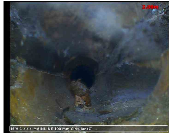
20211118-121754-snap0001.jpg, 00:00:24, 2.09 m Finish node, manhole, reference: MAINLINE - M/H2
