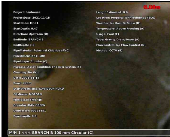
20211118-111716-snap0000.jpg, 00:00:02, 0.00 m Start node, manhole, reference: 1
