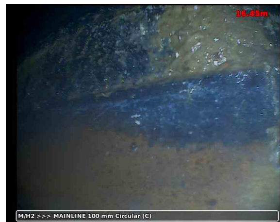
20211118-122831-snap0003.jpg, 00:02:11, 16.45 m Finish node, manhole, reference: 18
