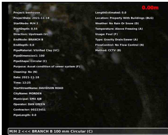
20211118-122550-snap0000.jpg, 00:00:02, 0.00 m Start node, manhole, reference: 2
