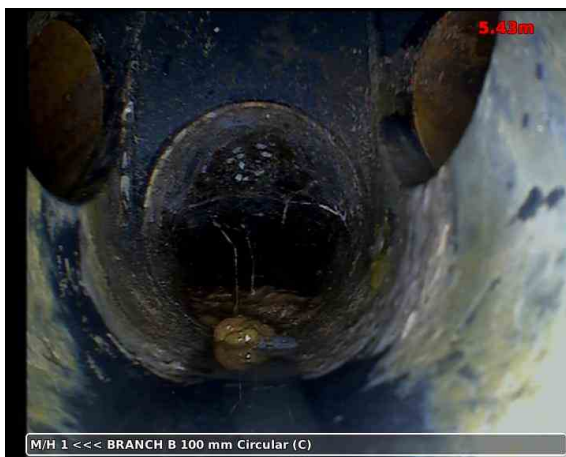
20211118-111716-snap0002.jpg, 00:00:51, 5.43 m Finish node, inspection chamber, reference: BRANCH B - INSPECTION CHAMBER
