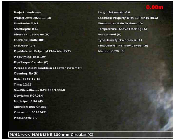
20211118-121526-snap0000.jpg, 00:00:02, 0.00 m Start node, manhole, reference: M/H1
