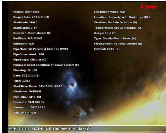
20211118-121754-snap0000.jpg, 00:00:02, 0.00 m Start node, manhole, reference: 1
