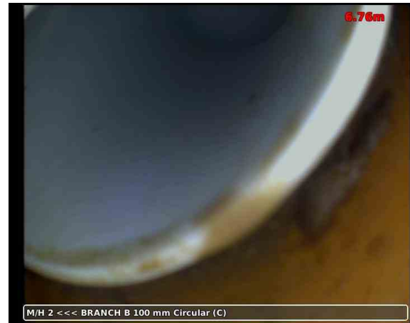
20211118-122550-snap0005.jpg, 00:01:37, 6.76 m Finish node, outfall, reference: BRANCH B
