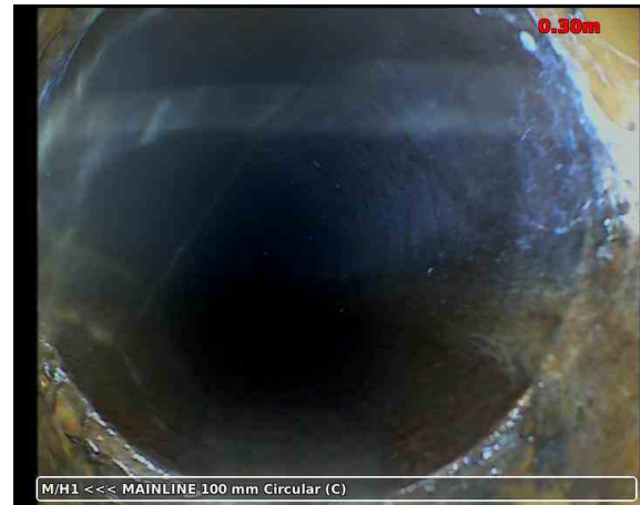
20211118-121526-snap0001.jpg, 00:00:27, 0.30 m Pipe material changes to vitrified clay at this point
